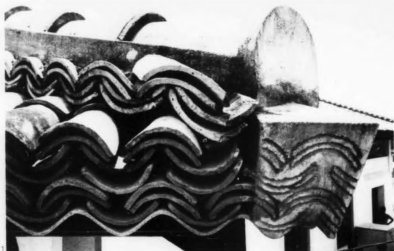
11, eaves detail used throughout. Bawa piles up the last few courses of tiles to get a thick, rich, ripply edge. The craftsmen suggested the decoration on the cement corners.
